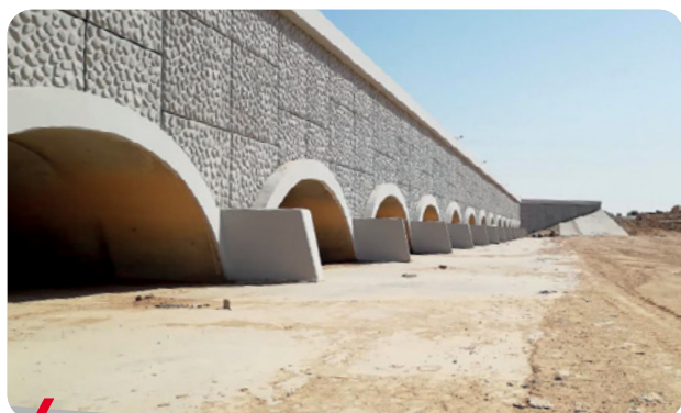
Wadi Stormwater Bridge, Saudi Arabia
