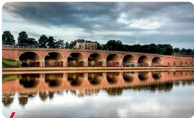
George Street Bridge, USA
